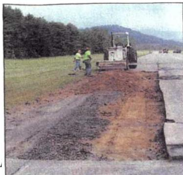
the subgrade, and replaced the base course prior to paving. A third crew expanded the north turn-around to better accommodate low-wing aircraft.
