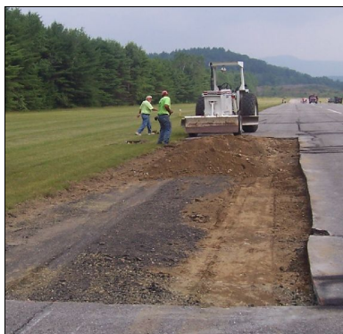
Repairs to a failed section of the runway.
