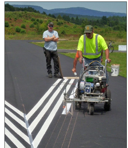
Painting an arrowhead for the displaced threshold.
