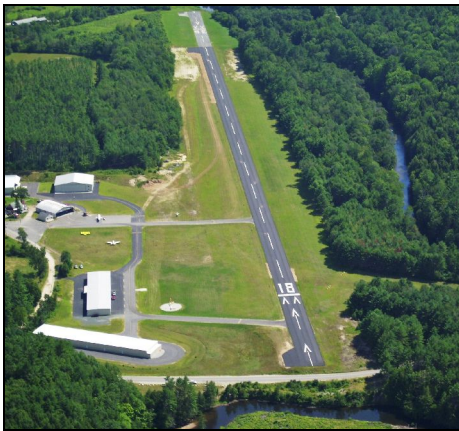
Looking south along the resurfaced runway with new markings for runway 18.
